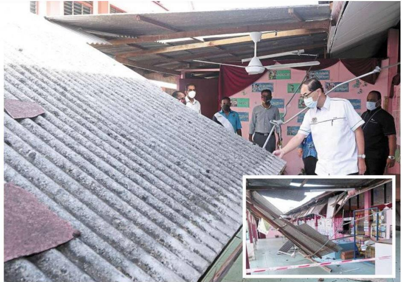
Inspection: Dr Mah inspecting the damage. (Inset) The fallen roof.
